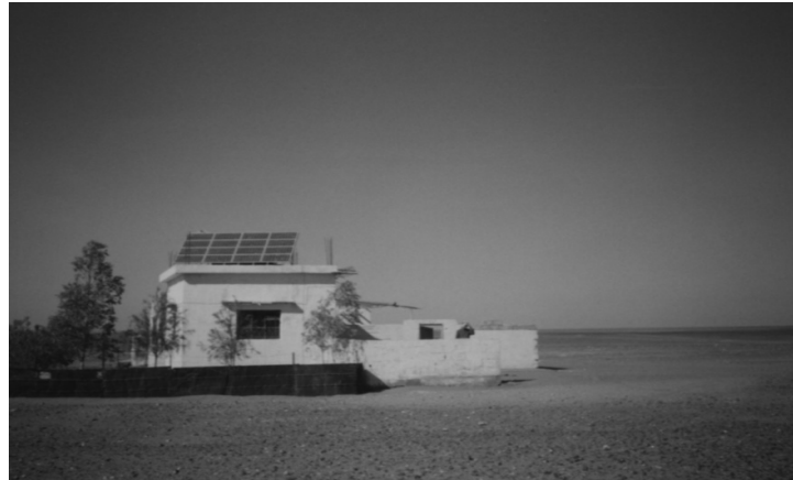
Figure 3. A household in Rawdet elnabdan village with the installed SHS on its roof.
