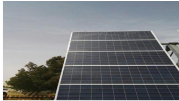
Figure 1. Serial One String Installation of PV modules
